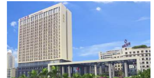
Foshan Fuxing Chancheng Hospital, China
